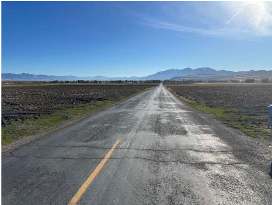
Figure 2 – 6400 West looking south along property frontage.
